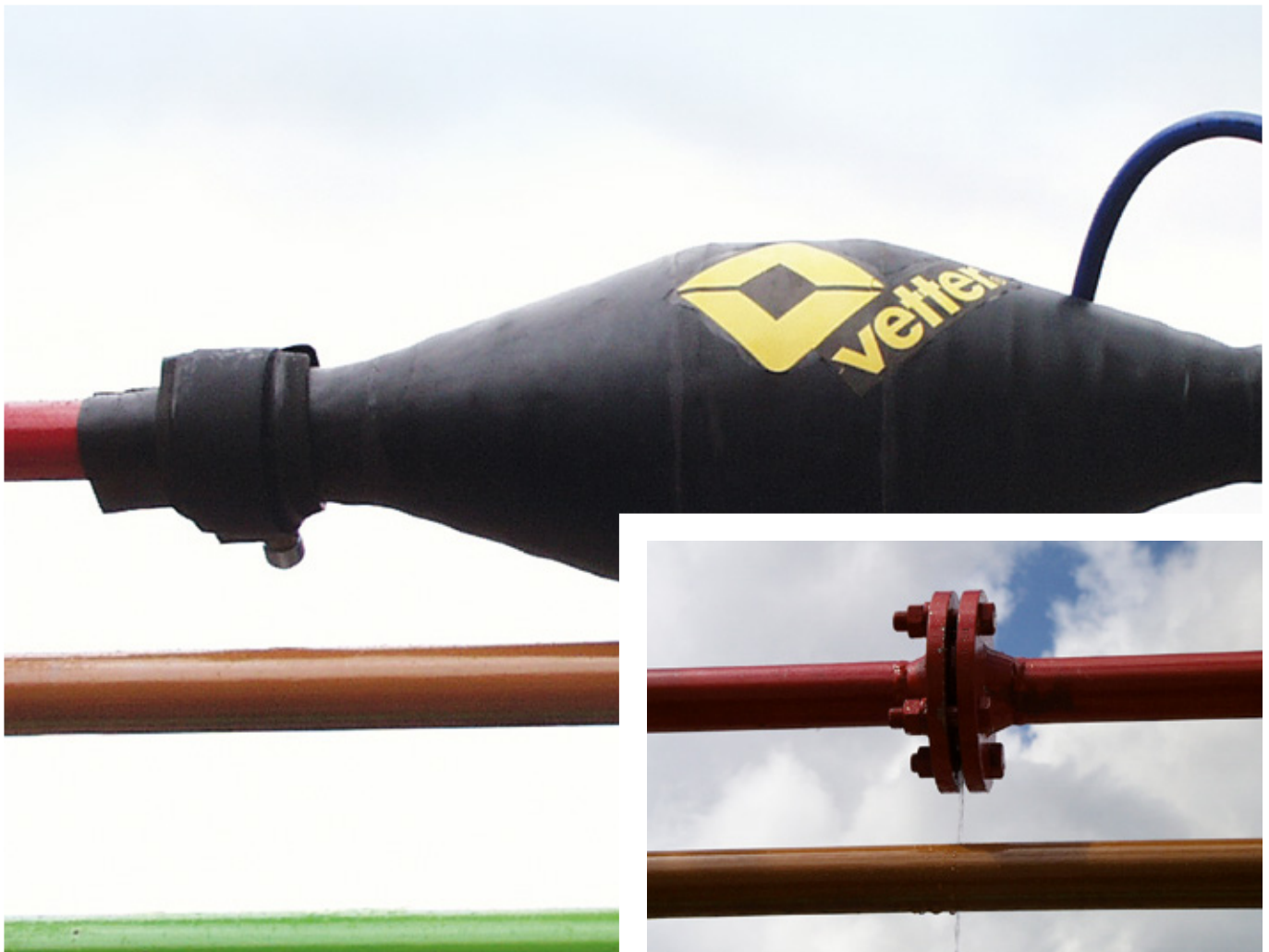
Leak in a pipe flange
