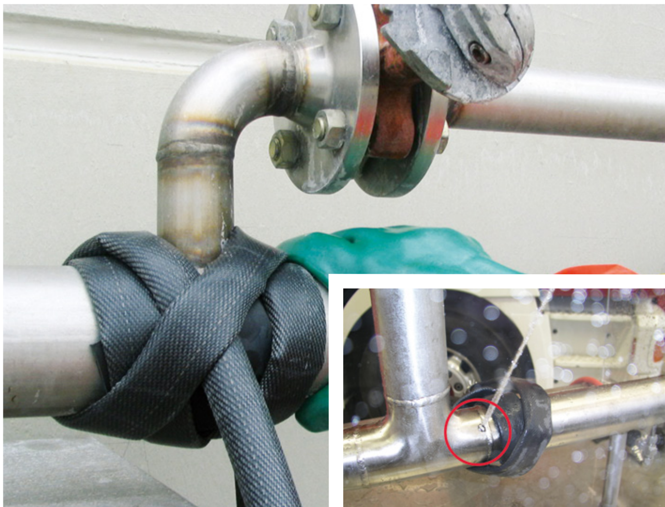
Precise-fitting sealing of difficult leaks
