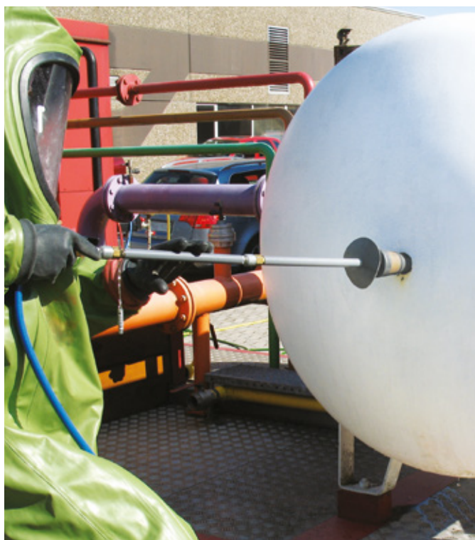
Seal leaks from a safe distance
